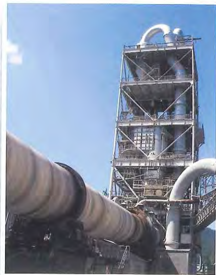
プレヒータとキルン New suspension pre-heater and Rotary kiln
